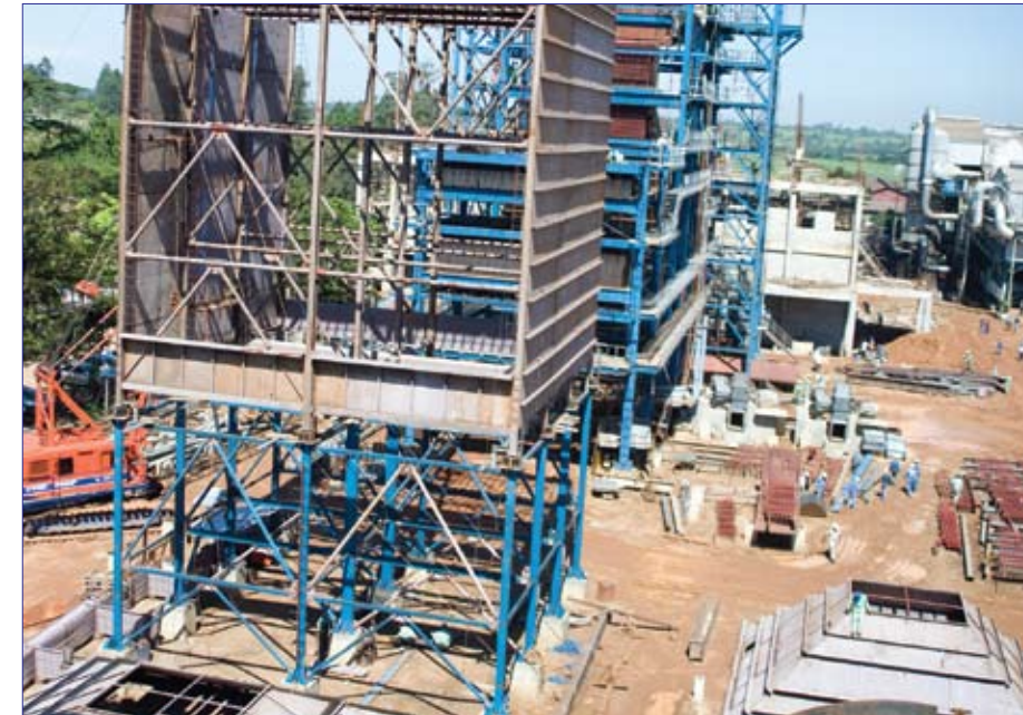
CoGeneration high capacity boiler under construction
