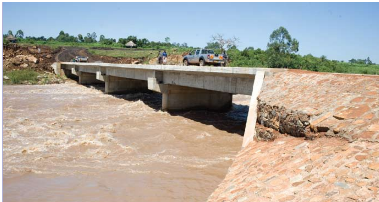
Matawa bridge on river Ng'oria nearing completion
