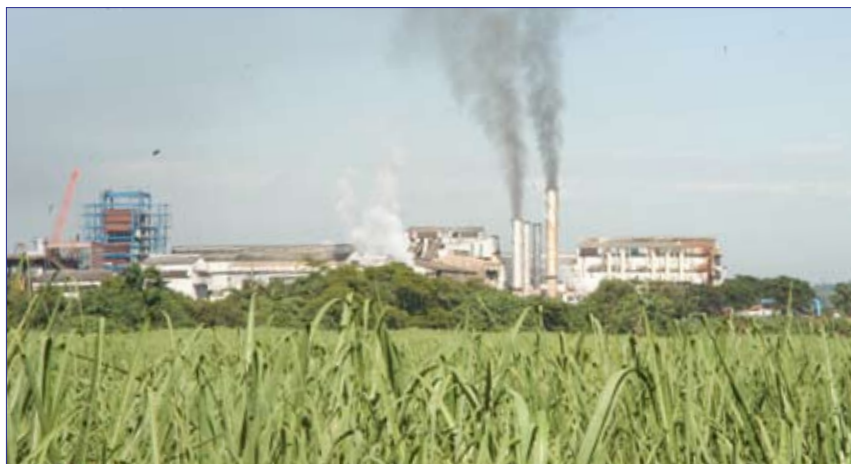
A rear view of the factory from the nucleus estate
