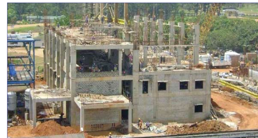
CoGeneration power house building under construction
