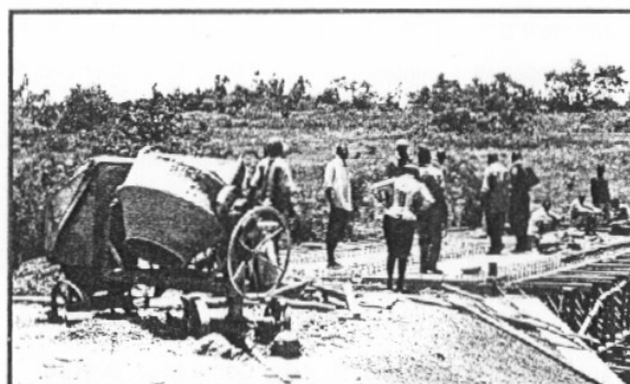
Bridge under construction
