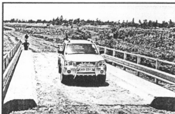
Bridge constructed by MSC to reduce cane transport distances
