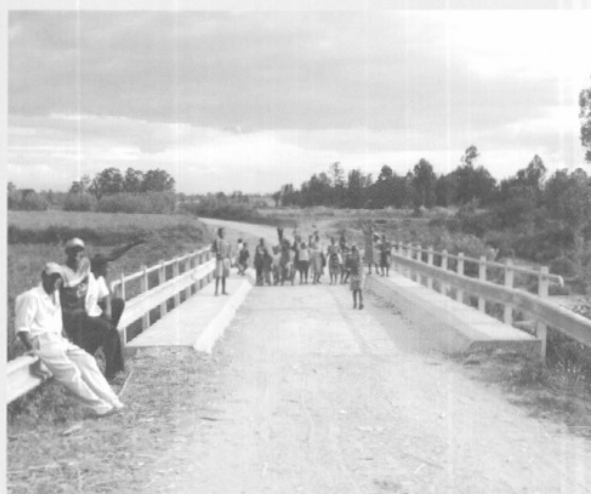
Lusumu bridge constructed by the company.
