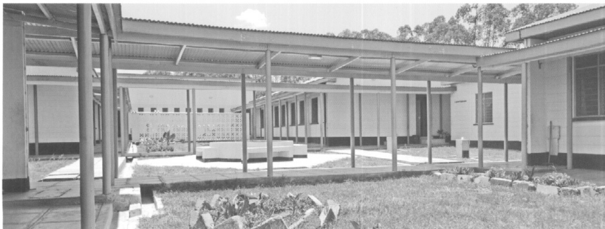
New classrooms built at Booker Academy.
