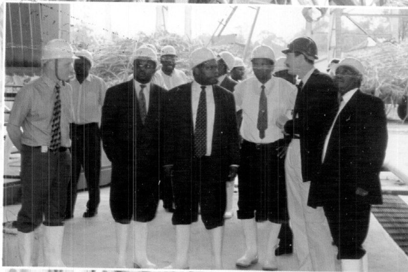
Directors on a tour of the ongoing construction aimed at upgrading milling capacity
