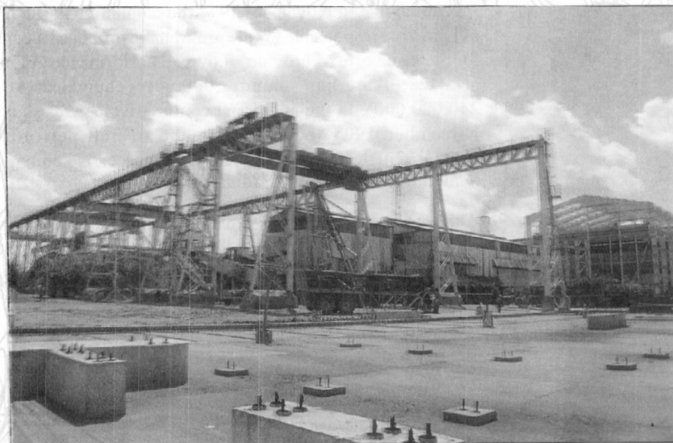
Expansion project under construction. The project is due for completion in 1997.
