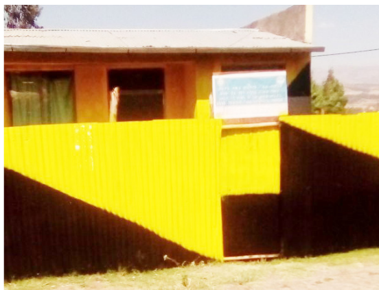
► Roto Ethiopia renovated the community police station
