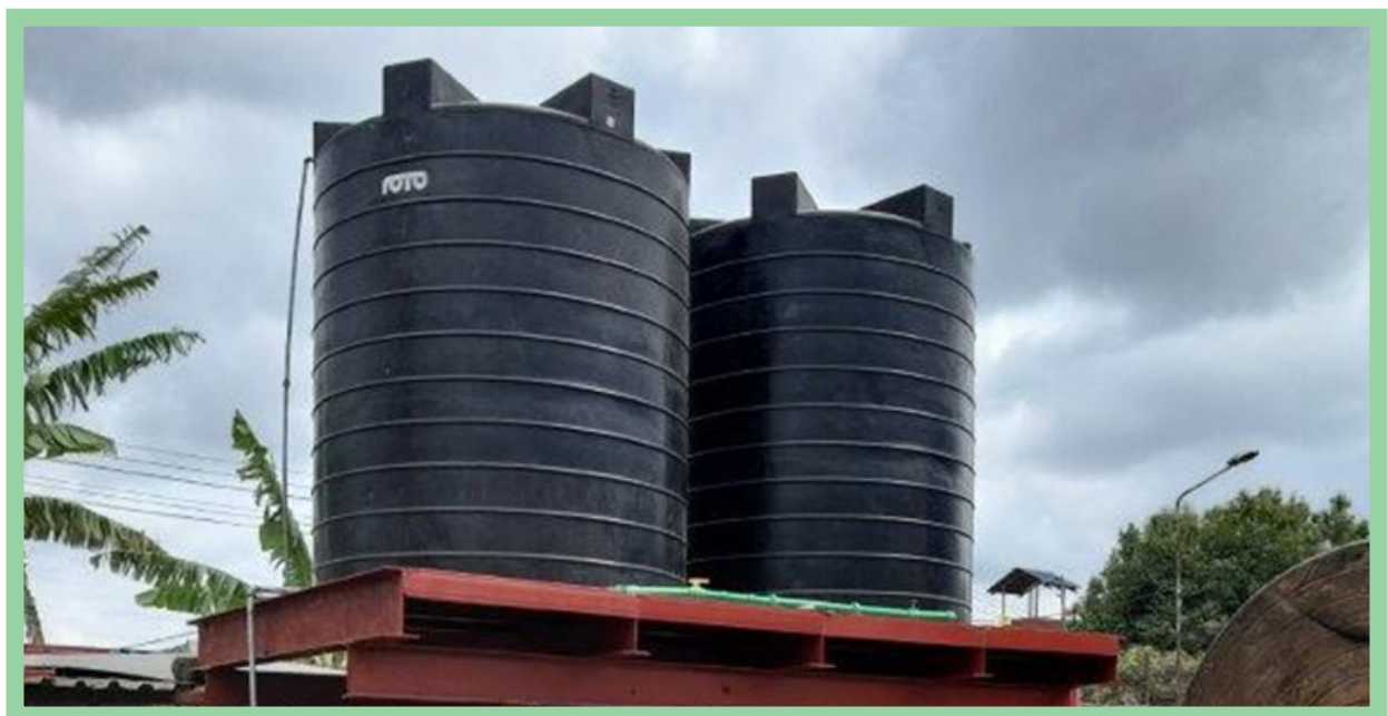
Constructed a water tower
