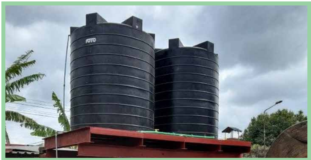
Constructed a water tower
