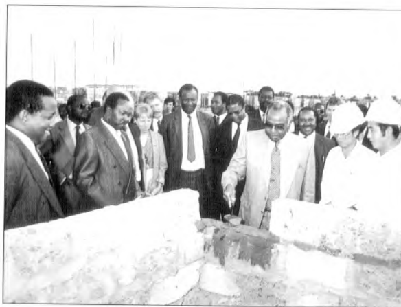
The Chairman Dr. B.M. Gecaga C.B.S. laying the foundation stone of the Imara Daima housing project.
