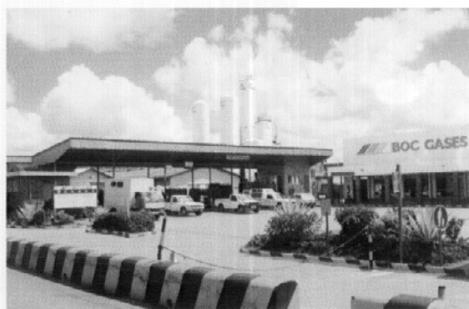
BOC Kenya Head Office situated along Kitui Road in Nairobi's Industrial Area.
