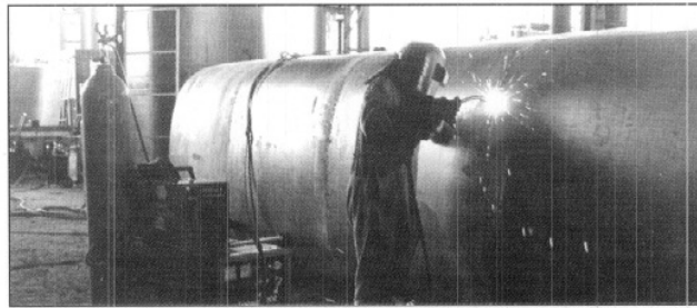
Arc welding in a steel fabrication industry using BOC Kenya products.
