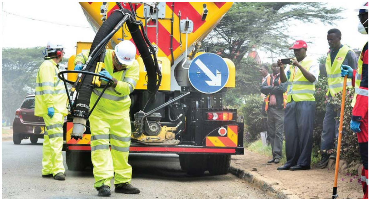
AEA a subsidiary of TC has invested in new technology that cuts the cost and time of road repair significantly.
