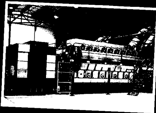
Tsavo Power Plant
