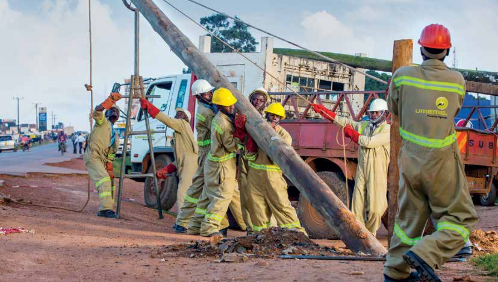
Mityana service crew manually erects a pole as part of their routine Maintenance
