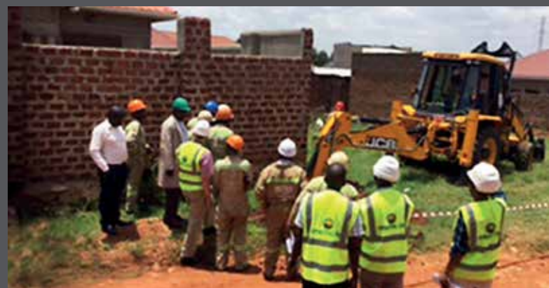
Nakulabye service crew replaces an old pole using the JCB vehicle which can replace up to 20 poles a day.
