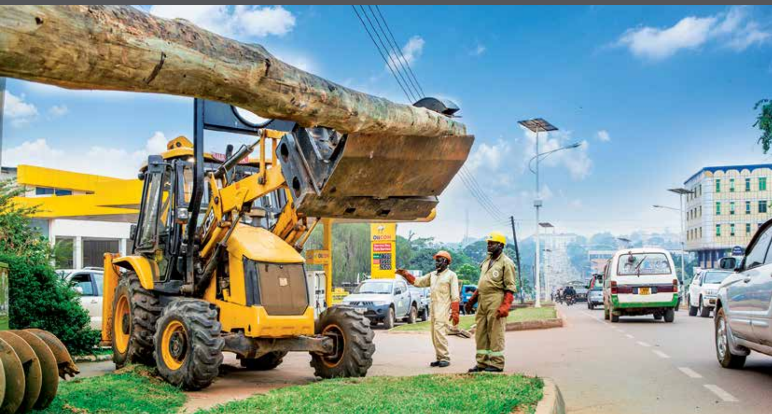
Nakulabye service crew replaces an old pole using the JCB vehicle which can replace up to 20 poles a day.
