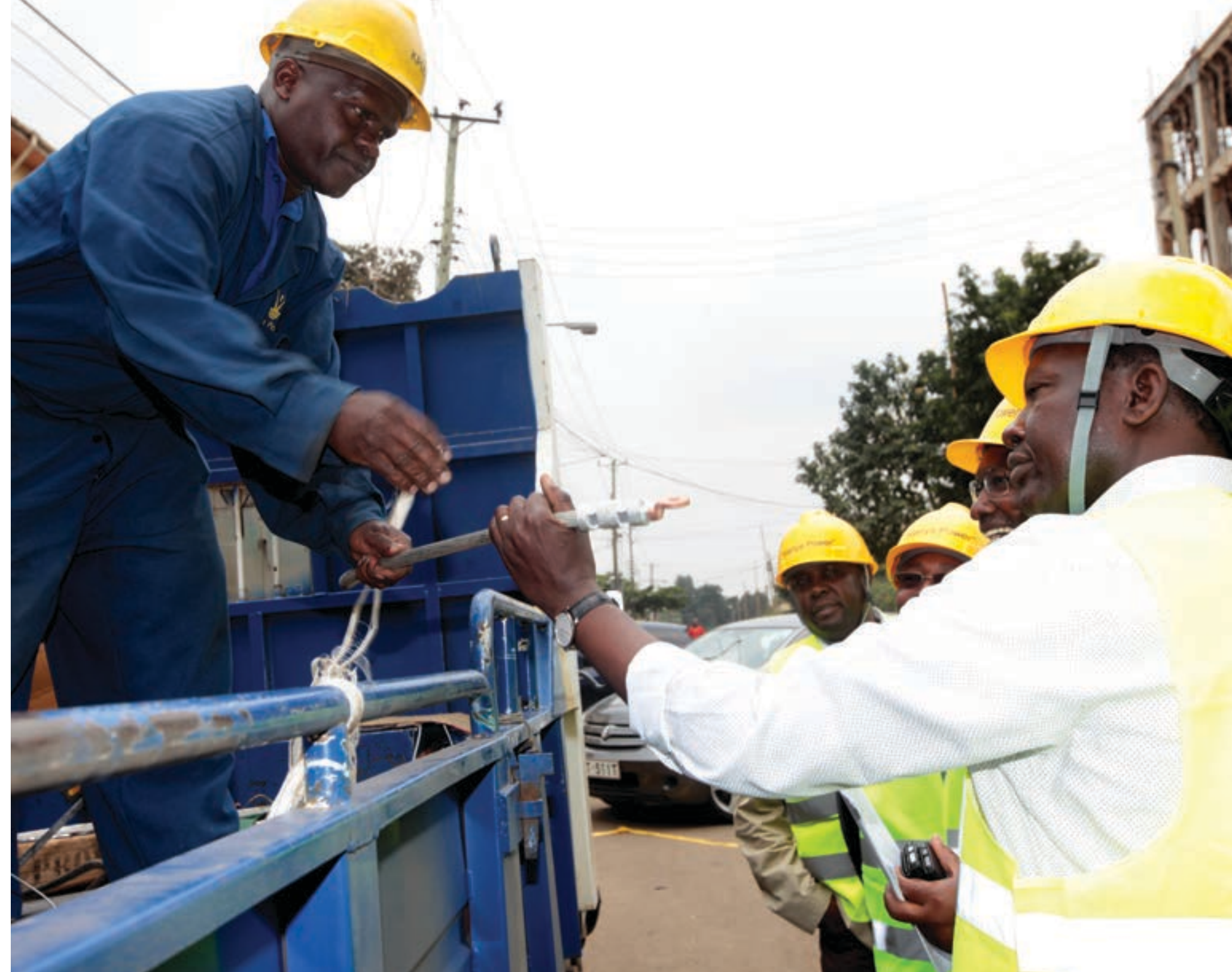
The Cabinet Secretary for Energy and Petroleum, Mr. Davis Chirchir, inspects an electric cable during a Boresha Umeme programme in Nairobi
