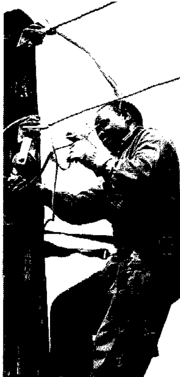
Line construction in progress
