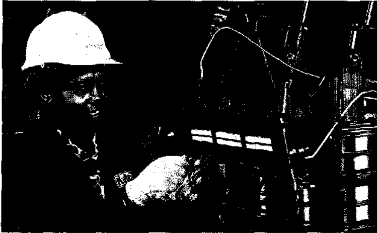
Final checks on electrical equipment before installation
