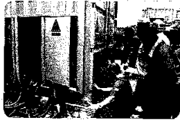
The emergency generators installed last year were decommissioned after water at the main Seven Forks dams improved, enhancing hydro-power generation.
