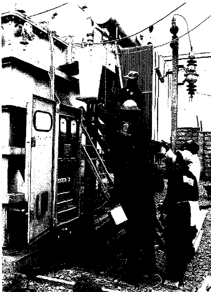
Constructing the new Kileleshwa Sub-station
