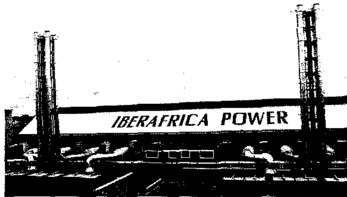
One of the two Independent Power Producers contracted to supply power to the KPLC, Iberafrica Power (EA) Ltd., installed a 44.5 MW diesel power plant at Nairobi South. It started commercial operations in June 1997.
