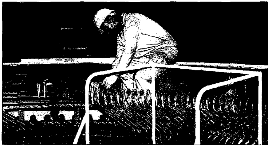
Major repair work on the 72.5 MW Gitaru unit No. 2 was completed and the unit put on load in January 1996
