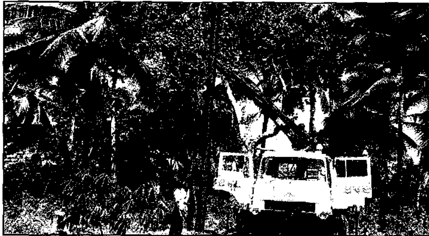
The Company embraced the move to liberalise the power sub-sector and contracted a private firm, Eve Africa, to construct the 61 km long 33 kV Kilifi-Malindi line
