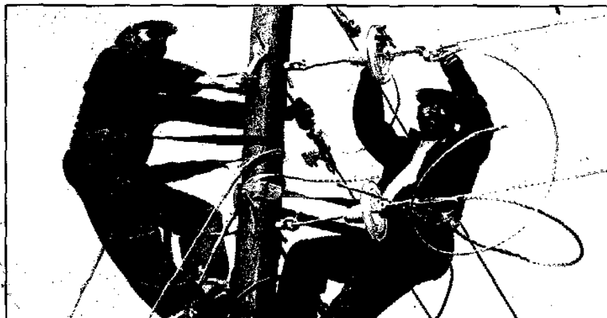
A rural electrification team strings a power line during the on-going electrification of Konza area in Machakos
