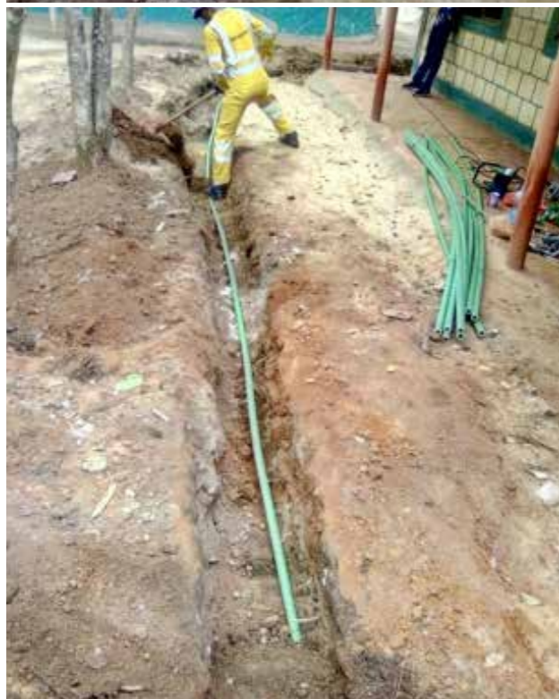
Installation of water pipes at Mkokoni Primary School - Kwale County.
