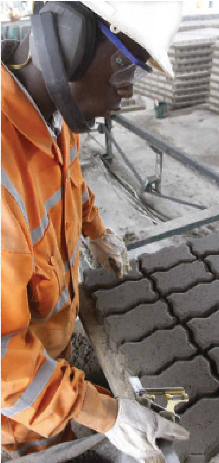
Employee making concrete blocks
