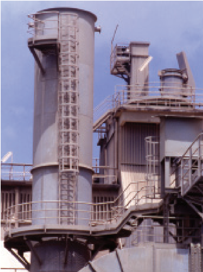
Rotary Kiln 1 stack at Mombasa Plant
