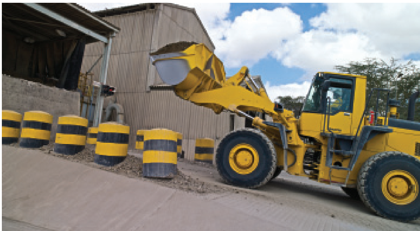
Wheel-Loader feeding the additives belt at the Nairobi Grinding Plant
