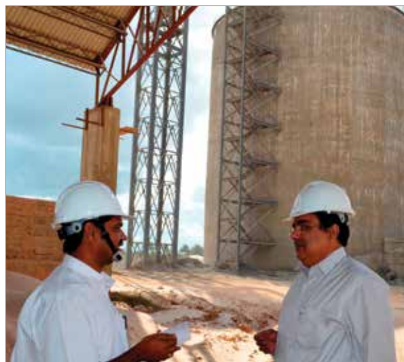
Deputy Managing Director Surendra Bhatia, with Dar es Salaam cement plant General Manager Girish Kumar. In the background gypsum storage building and 15,000 ton capacity clinker silo.
