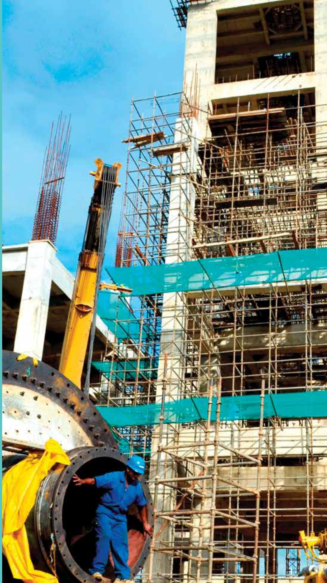
Mechanical erection at the 4,000 tons per day Clinker plant at Tanga.
