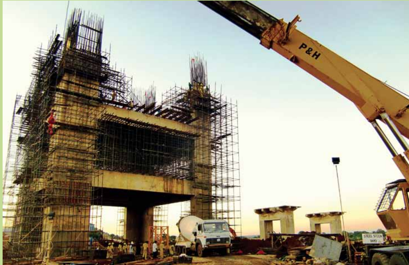
INSULATION OF HOT GAS DUCTING AT KALOLENI PREHEATER TOWER AND PREHEATER TOWER UNDER CONSTRUCTION AT TANGA
