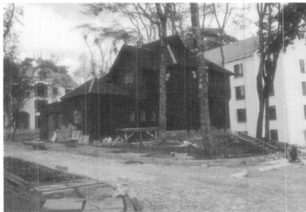
GETRUDES GARDEN DEVELOPMENT, 40 HIGH CLASS APARTMENTS ON MUTHAIGA ROAD, DEVELOPED BY A PARTNERSHIP OF GETRUDES GARDEN HOSPITAL TRUSTEES AND THE BANK'S PENSION FUND. THE DEVELOPMENT INCLUDES RESTORATION OF THE ORIGINAL WOODEN GROGAN HOUSE (FOREFRONT)
