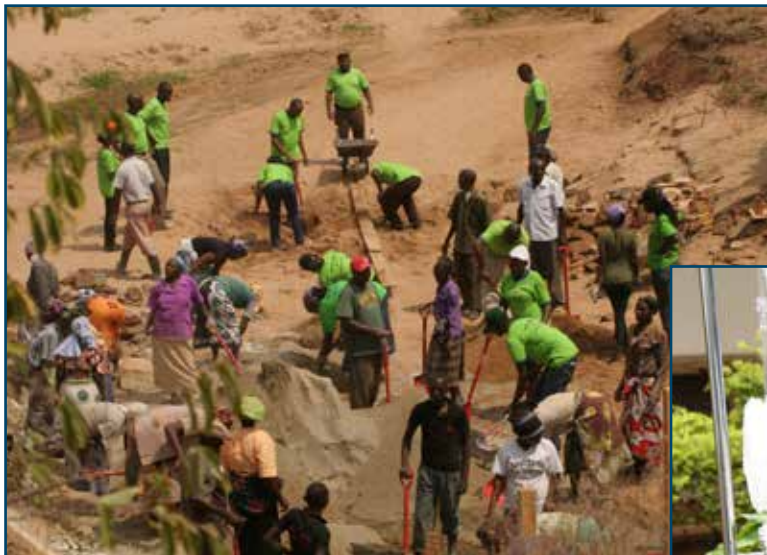
Staff members during the construction of a sand dam along river Thange in Kibwezi District, Makueni Constituency. The dam, constructed by KCB Foundation in partnership with Africa Sand Dam Foundation will benefit members of Wendano wa Mambo Group to gain access to clean water for domestic and farming use.
