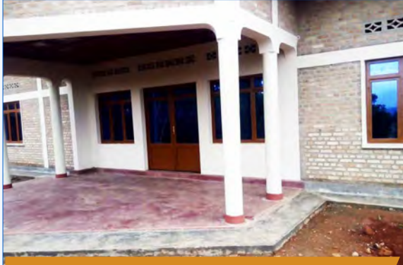
One of the houses constructed by AVEGA-AGOHOZO with the sponsorship of BK
